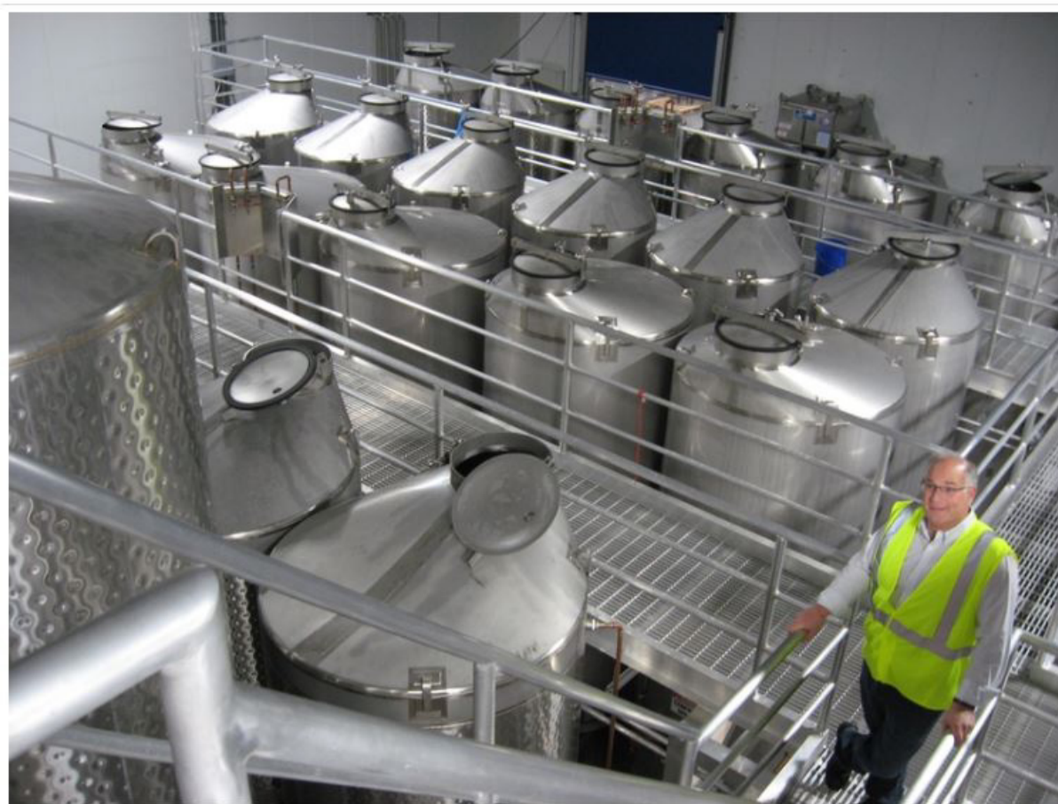
COO Rich Bouwer in the Free Flow wine cellar where 50 tanks and 30 portable tanks store wine to be kegged or canned.
